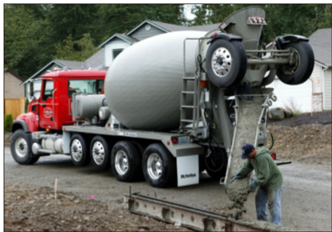
Concrete being poured into a form.
